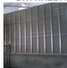
Board joints are staggered
